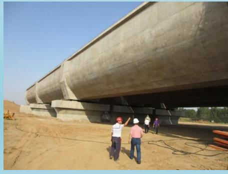
Duan he flum, length 1030m, discharge 350m<sup>3</sup>/s, increase discharge 420m<sup>3</sup>/s
