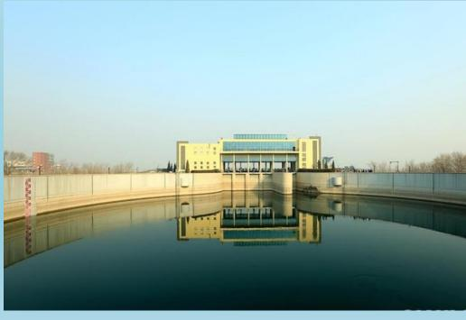
Daning pressure regulating pool, diameter 80m, depth 16m, volume 78000m<sup>3</sup>.
